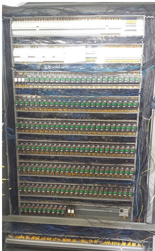
Figure 3. Example of Relays installation in sample case of automation system
